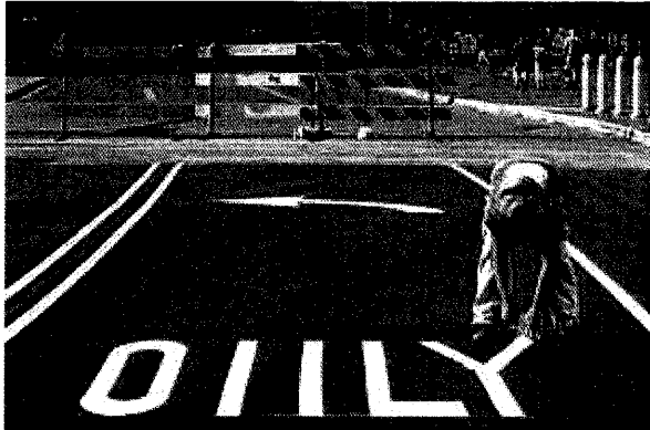
Zoom Kim Weiss positions markings in a left-turn lane on McCamly Street. / Kevin Hare/The Enquirer
