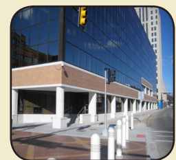
The facade renovation on 67 W. Michigan Avenue.
